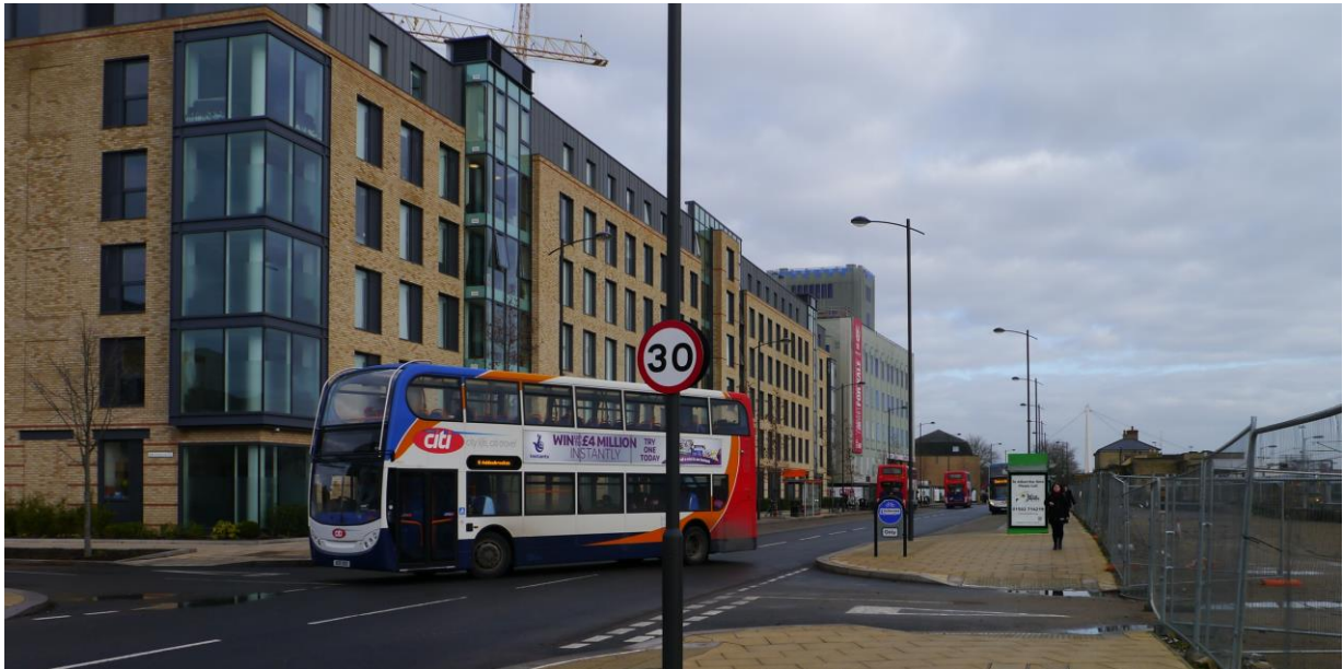
Bus interchange and redevelopment at Cambridge Station
