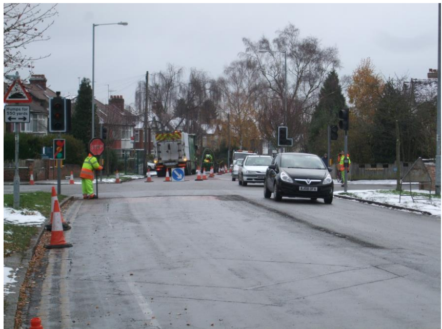
Construction of the Gilbert Road, Cambridge cycle lanes scheme
