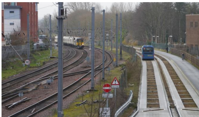
Rail and Busway corridor south of Cambridge station
